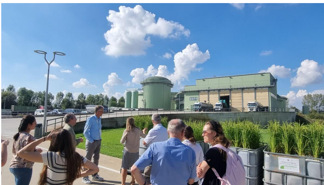
Aqua & Sole Sewage sludge treatment plant
